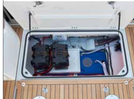
Storage below cockpit floor
